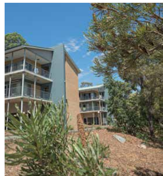
ECU Village – South West Campus
